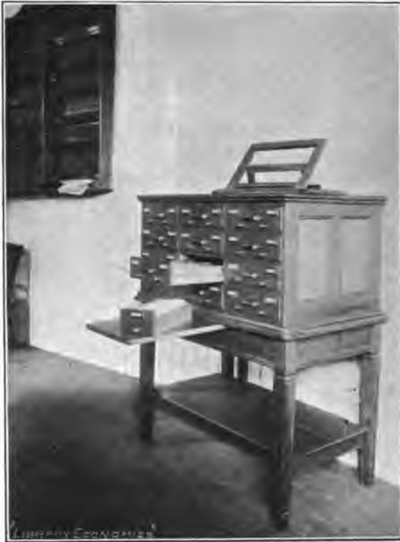
FIG. 115.—Card Catalogue Cabinet, with Sliding Extension Runners (Section 351).
